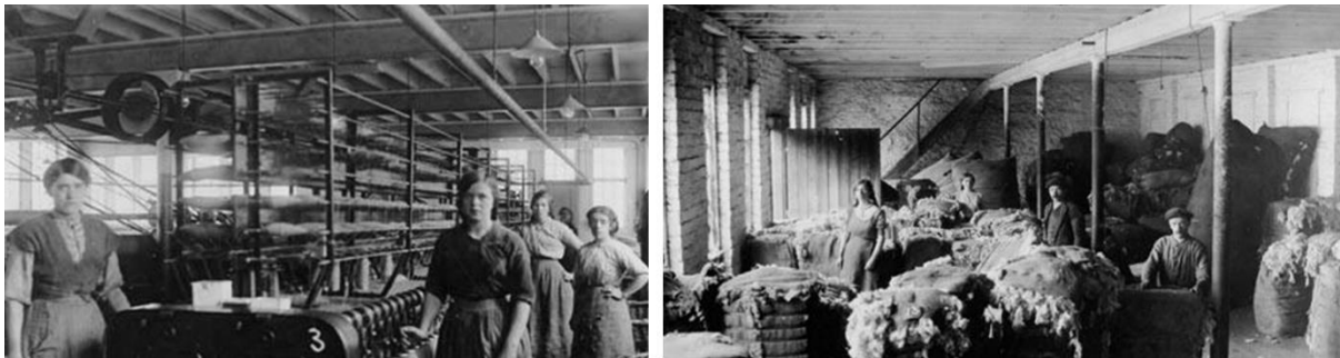
Figure 1 Blackwood Brothers' River Mill, Kilmarnock (Left) The floors were supported on cast iron structure ; (Right) beams were supported by hollow circular columns (East Ayrshire Libraries, 1917)
