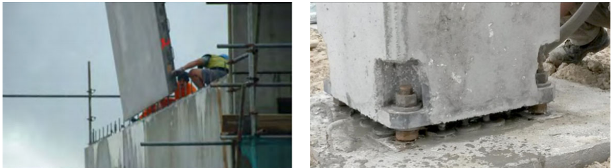
Figure 15 Grouted dowels (left), bolted steel plates (Engström, et al., 2008)
