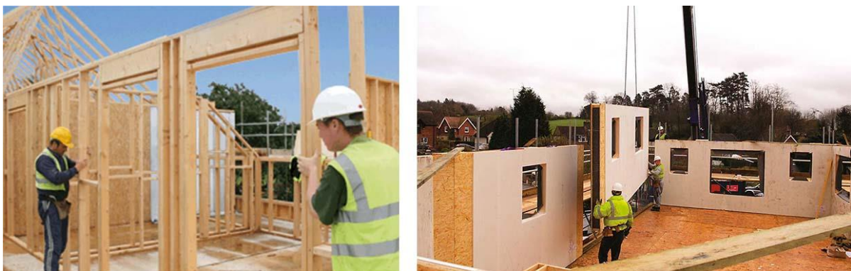
Figure 4 Timber Frame Systems; Open Panel System(left) and Closed Panel System(right)
