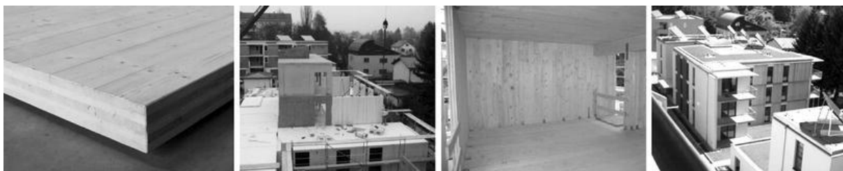
Figure 7 (Left) five-layer CLT element; (middle to right) impressions from project Wittenbauerstraße/Graz/Austria: two three-storey residential buildings
